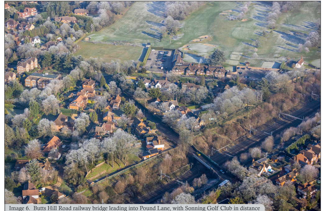
Image 6. Butts Hill Road railway bridge leading into Pound Lane, with Sonning Golf Club in distance
