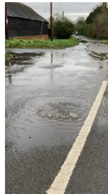
Thames Water pumping station ineffective
