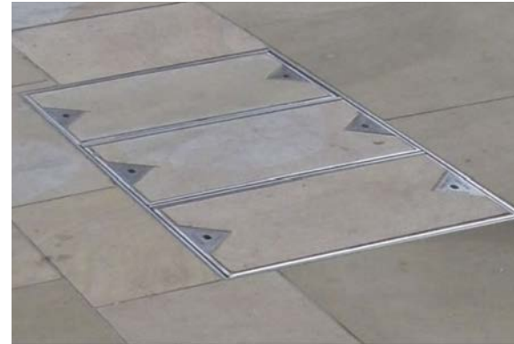
EXAMPLE OF A RECESSED INFILL SERVICE COVERS
