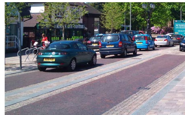
EXAMPLE OF WIDE CHANNEL LINE AND HOW HOT ROLLED ASPHALT CAN BE USED TO IMPROVE CONTINUITY IN MATERIALS ACROSS THE STREET
