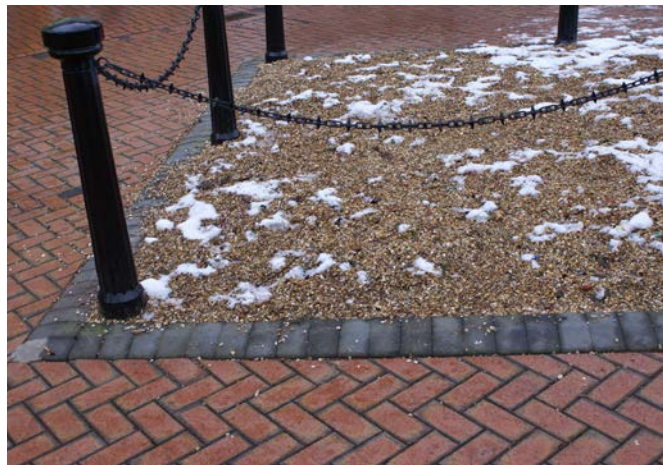
PAVEMENT HEAVE CAUSED BY TREE PLANTING
