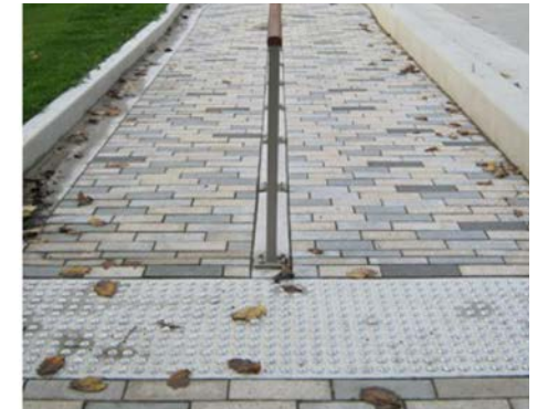
TACTILE PAVING IN MATCHING/COMPLEMENTARY MATERIALS
