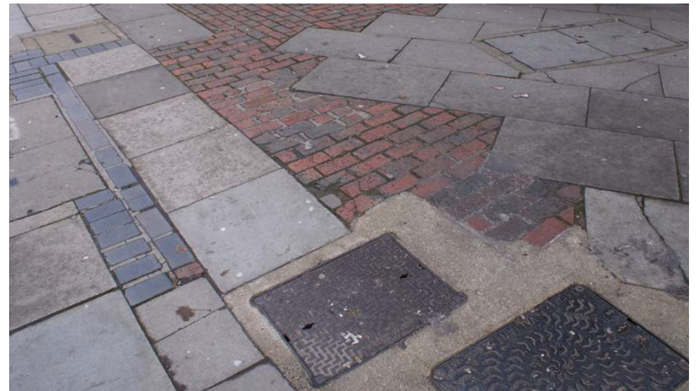
TOO MANY PAVING MATERIALS, POOR REPAIRS, UNEVEN SERVICE COVERS
