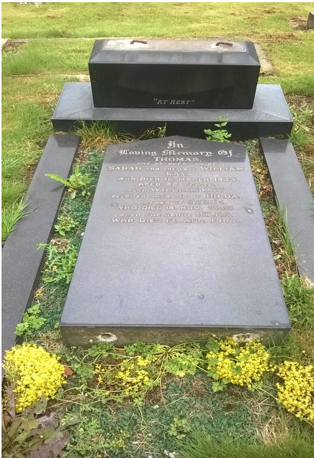
Example of an unsafe memorial laid flat in between existing kerb sets
