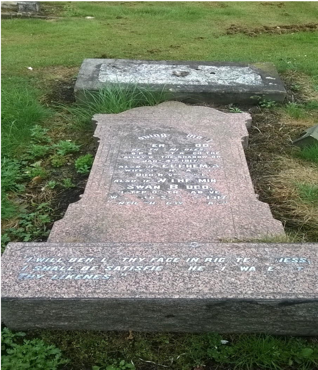
Example of an unsafe memorial, with no dowels, laid flat on the existing grave space.
