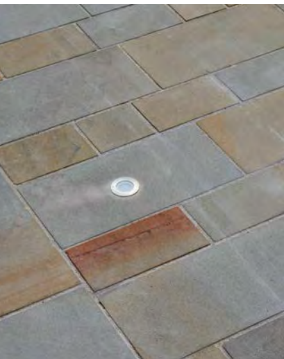
Yorkstone paving – Versatile material allowing features to be cut into it and specified to a range of sizes
