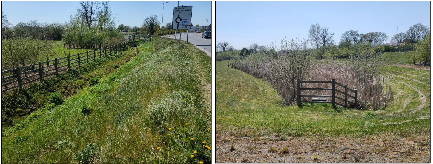
Figure 9-2: Examples of SuDS along Shinfield Relief Road (Swale (left) and Wetland Basin (right))
