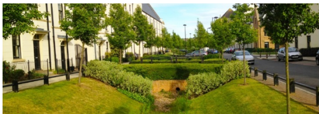
Swale: Shallow, grassy channels designed to store storm water run-off
