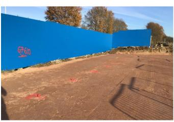
The installation of Network Rail asset protection hoarding has been completed, allowing us to work safely to complete the piling platform. Also, the setting out of the 28No. piles has been undertaken, ahead of the piling works.
