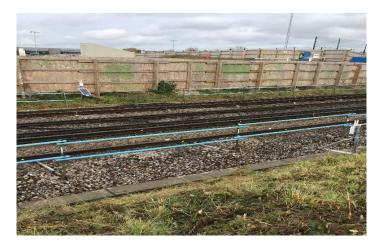
Vortok fencing and track monitoring devices have been installed on the rails along the track to enable the works in preparation for the new bridge over the railway.
