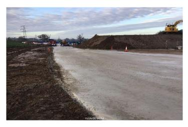
The majority of the stabilised haul road has now cured and is ready to use after achieving bearing capacity of over 500kN/m2.
