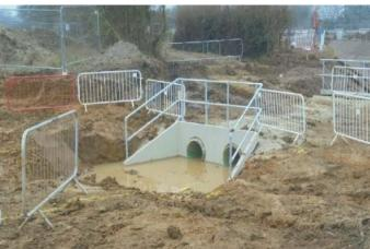
The last of the precast headwalls of the new stream has been installed
