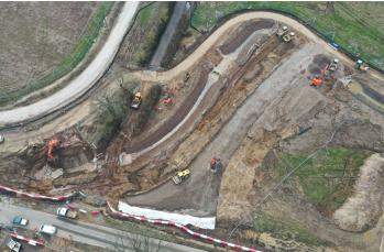
Aerial view of Waterloo Road site works. Work is being carried out to construct a new stream that will better manage the water in this location, work on the southern arm of the roundabout is also being carried out.
