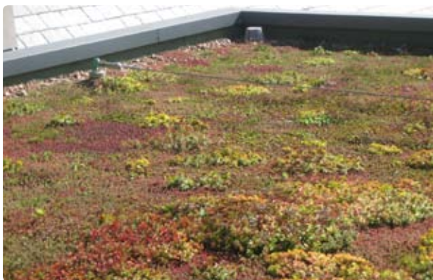
In Exeter a modern extension to a listed mill building utilises a low maintenance sedum roof that minimises rainwater run-off and provides a valuable city centre habitat.
