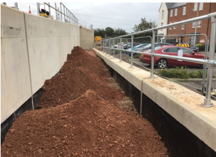
Above Left photo shows the wheelchair access ramp being constructed along the wingwall.
