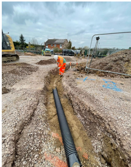
Works ongoing to install new drainage and kerbs at both sides of the new road that links into Bell Foundry Lane.
