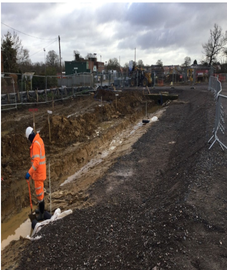
Works ongoing to install new drainage and kerbs at both sides of the new road that links into Bell Foundry Lane.
