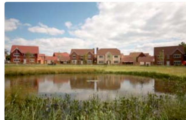
Sustainable Urban Drainage principles have been built into the layout of The Carillons, Wokingham providing a strong setting for development and an important open space network.
