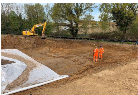
Works are progressing at former allotment site next to the BP Garage on the main Reading Road in readiness for the bridge abutment works.
