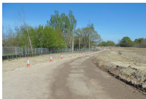
Temporary haul road which runs from Old Forest Road will enable easier access during main construction.
