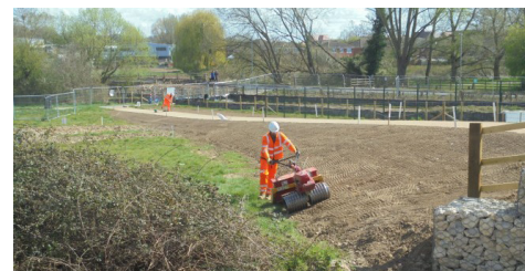
Shown here is BLEC machinery, a fast and effective way of seeding all areas. The low ground pressure exerted by the Cultipack Seeder makes it particularly effective on sensitive ground.
