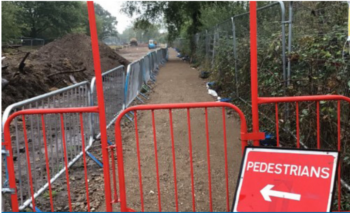
Winnersh Relief Road safety measure: A temporary pedestrian walkway has been installed through the northern roundabout site. This helps to create a visual exclusion zone between plant and pedestrian
