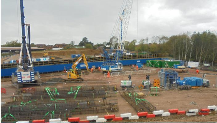
The piling rigs are assembled and reinforcement steel prepared
