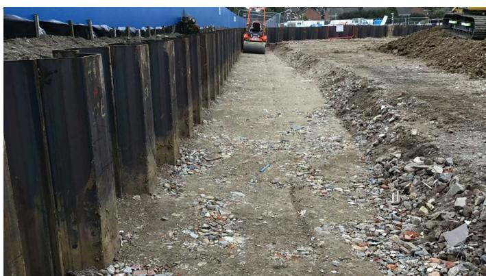
Sheet piling installation completed. The system will protect the railway during the new bridge piling work
