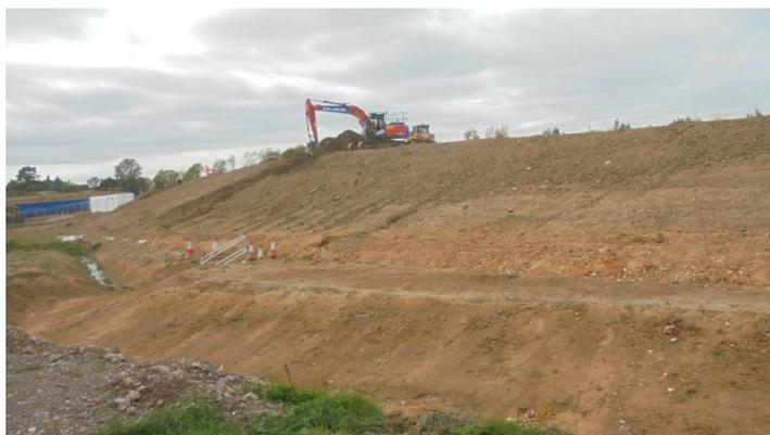
Finished embankment leading to the new railway bridge. The embankment is 8m higher than the original ground. The finished level of the embankment is expected to be at the same level as the M4 as this is the height required to clear the railway
