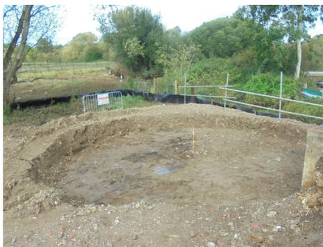
Ground preparation for caissons which will be used for the foundation of the new footbridges in the Emmbrook watercourse
