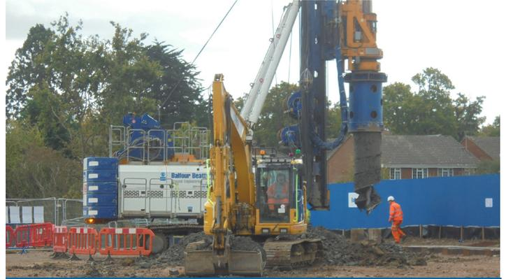
Rotary excavation for the piles is progressing. Piling work is taking place on both sides of the railway simultaneously. The tall blue cranes can be seen from the Reading Road and surrounding area
