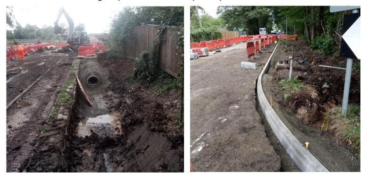
Photo above Left: New drainage system being installed in at the Park Lane/Nine Mile Ride junction. Photo above Right: The new kerbs being installed to the new levels at the Park Lane/Nine Mile Ride junction.
