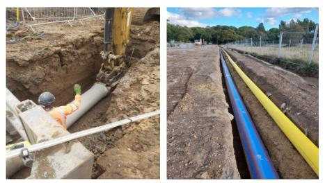
Photos on the left: Show underground drainage and utilities materials being installed.
