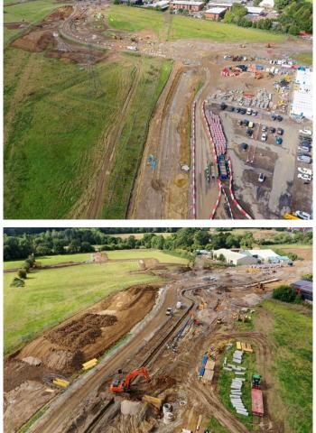
Main construction works are well underway at a number of locations across the sites, focusing initially on the bulk earthworks and drainage works as well as working with the utility companies to install and divert all the necessary services such as gas, water and electricity. As you can see, works have progressed to the extent that the beginnings of what will become the new road alignment are starting to take shape on the ground.
