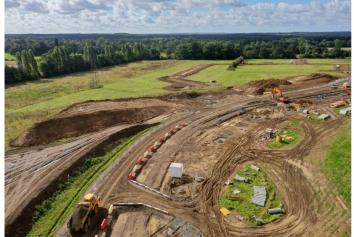
Photo on the right shows works at the junction of Park Lane/Nine Mile Ride. These works included install of new drainage systems, connection of new utility supplies to existing supplies and tiein of the new road to the current junction. The junction was reopened at the end of October 2021.
