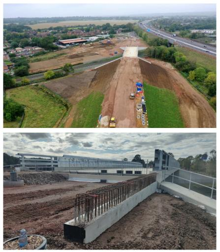
Works are still continuing at pace on and around the New Railway bridge. Photos on the left and below show the "backfill" operation continuing to be carried out to link the bridge structure to the new road. During the backfilling, the soil is compacted back into the foundation. The bridge deck and parapet works have already been completed. The "backfill" works are planned to be completed by end of October 2021, and the final road and footpath surface should be in place by early 2022.
