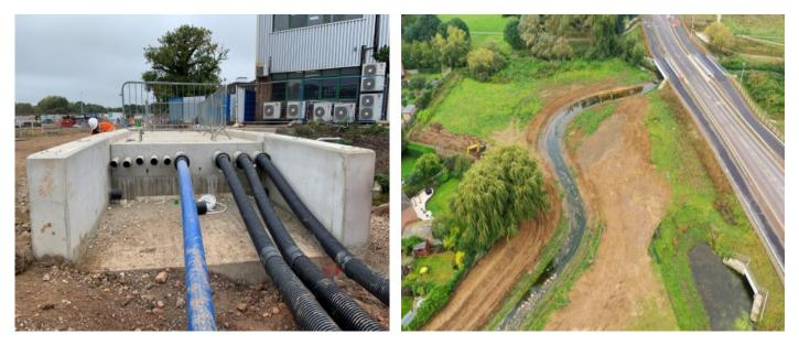
**Photo top left:** New utility supplies being installed through the new walkway/bridge at Toutley Road.
