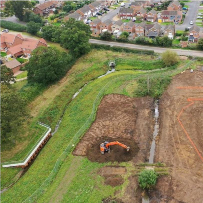
Works to divert the Ashridge Stream into a culvert under the route of the new road were recently completed. Nearby trees were protected to prevent damage during construction of the road and works on the two new ponds north of the road have also been completed. Not only will these take all the run off from the road, but they will also create a new habitat for local wildlife.
