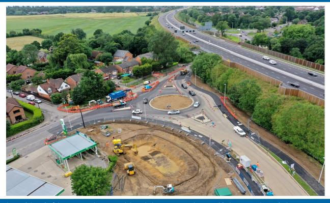
Aerial view (above) of the new Southern roundabout linking onto Reading Road (adjacent to the M4), this is now open to traffic. Pavement construction has started at the south roundabout, the install of the drainage and service ducts has now been completed.
