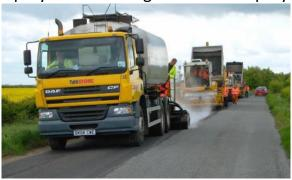
**Stage 2** – Stone chippings are applied to the top of each layer.
