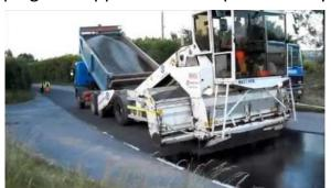
**Stage 3** – The chippings are then rolled to press the stones. Once the road is open, the moving traffic further embeds the chippings.
