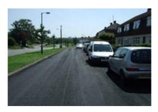
**Stage 4:** When the chippings have bedded in, we sweep the road two or three times to remove the excess chippings and refresh road markings if necessary. This can take up to two weeks.
