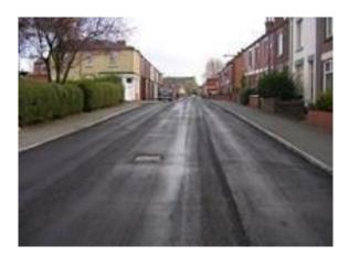
**Stage 3:** When the road has fully stabilised the white and yellow road-markings will be remarked. Any ironwork lower than the new road surface will be broken out and raised or replaced. Once the concrete bedding and surround is ready, the operatives will reinstate the surfacing with microasphalt material. These reinstatements will blend into the rest of the surface with use.
