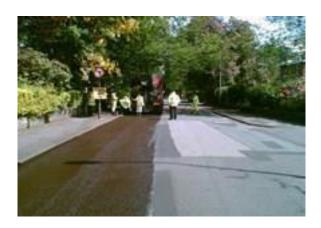
**Stage 2:** The micro-asphalt will be left to fully bed in for approximately three to seven days following which the road will be swept of loose material. The condition of the road will continue to be monitored with further sweeping being carried out on an ad-hoc basis as required.
