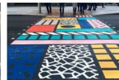
Thermo plastic markings applied to asphalt road surfaces in heavy trafficked area
