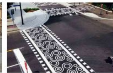
Painted markings on road surface using pattern to denote crossing points.
