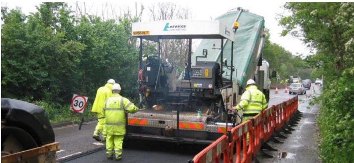
The above image shows a paving machine in operation. The hot material is delivered in insulated lorries – one is tipping into the front hopper of the machine in the picture – and the paver lays it in an even layer out of the back of the machine. Just visible in the corner of the photograph is one of the rollers used to compact the material after it is laid.
